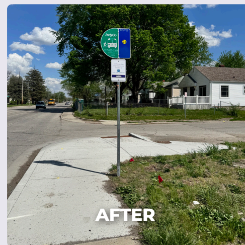
Above: the reconstructed ADA-accessible stop at North Linwood Avenue and East 21st Street. Changes include improved curb ramp, wider sidewalk and rider waiting space, and better drainage for longevity.
